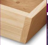
The set-up block is all you need to cut a perfect compoundangle butt joint. The block should be narrow enough to fit under the teeth of the blade when it is fully raised, with the end of the block flush against the blade's side.
